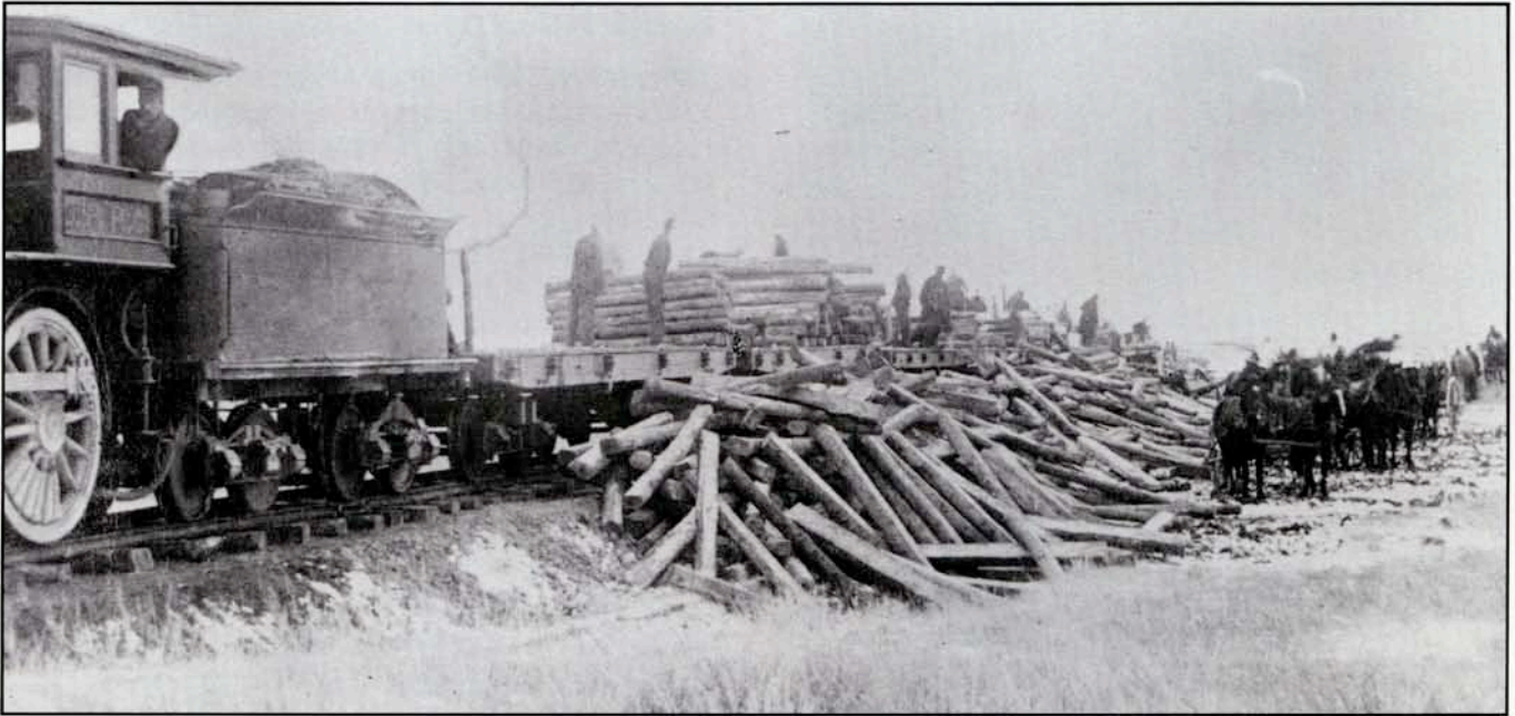
Unloading ties near Regina for railway construction, 1882-83.
